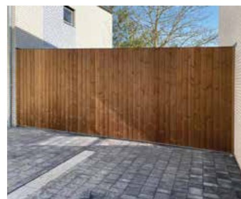
Thermowood verticale beplanking
