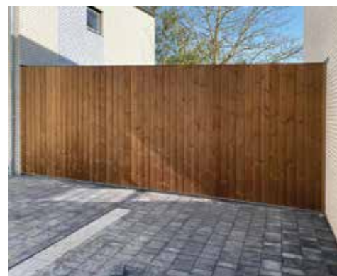
Thermowood verticale beplanking
