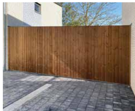
Thermowood verticale beplanking
