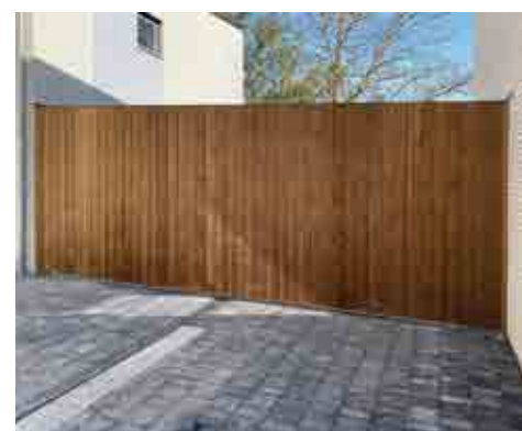
Thermowood verticale beplanking
