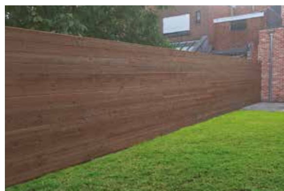
Thermowood horizontale beplanking
