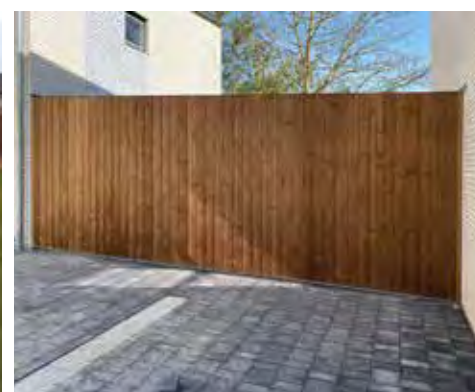
Thermowood verticale beplanking
